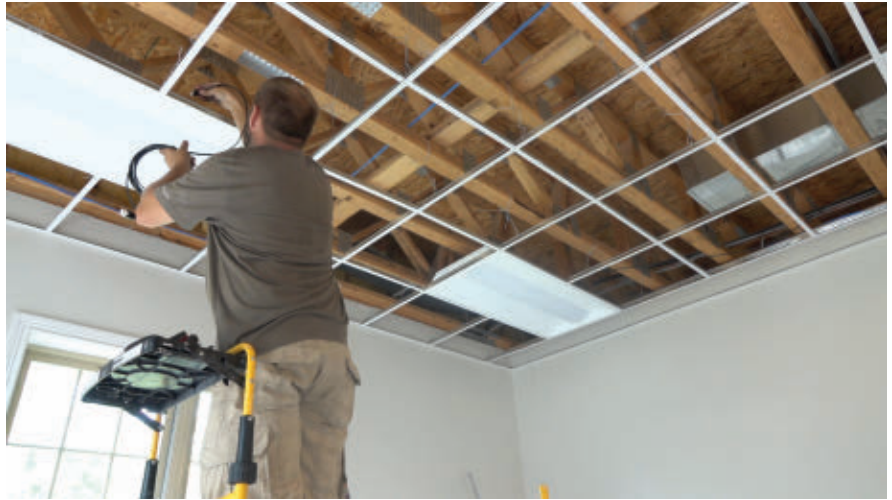
FIG. 4. The low-voltage cable connects directly to the luminaires in a DLVP system and a single DC channel can be daisy chained to multiple luminaires.
