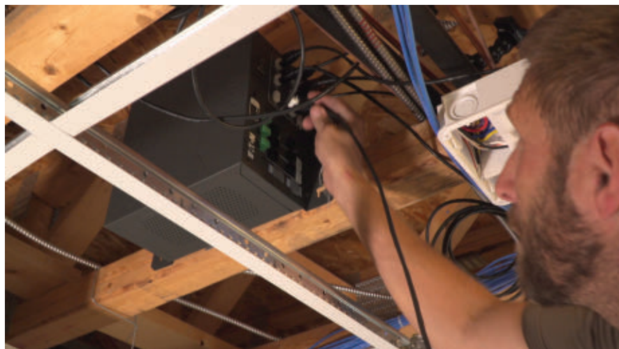
FIG. 3. Making the connection between the PDM and a luminaire is simple, and the cable is left exposed in the raised ceiling and secured with simple cable ties just like Ethernet cable.
