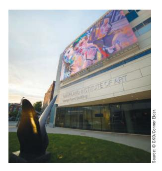
What sets the LED mesh display installations apart including the CIA work is the ability to make the SSL installation an integral part of a building's architecture while enabling dynamic images and even video content. Indeed, the GKD screen at the CIA is mostly transparent allowing natural light to enter windows behind the screen and and enabling people inside the building to see out. " page 10
