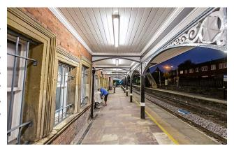
It was important to integrate new technology into the historic station without any detriment to the location. The lights previously installed on site included internal SON units, 6ft fluorescent fittings and HID external HID column top units. They were replaced with DEXECO's Impervia LED column, Hydra LED, MODLED and Amenity Plus LED.
